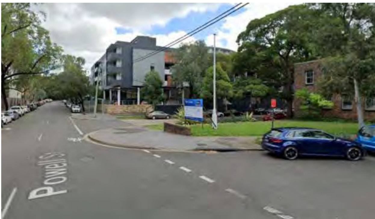
Photo 3: Powell Street looking west, with the apex of the site on the right, and sag point overflow point located at the end of the road. Source: Google Street View, dated March 2021.
